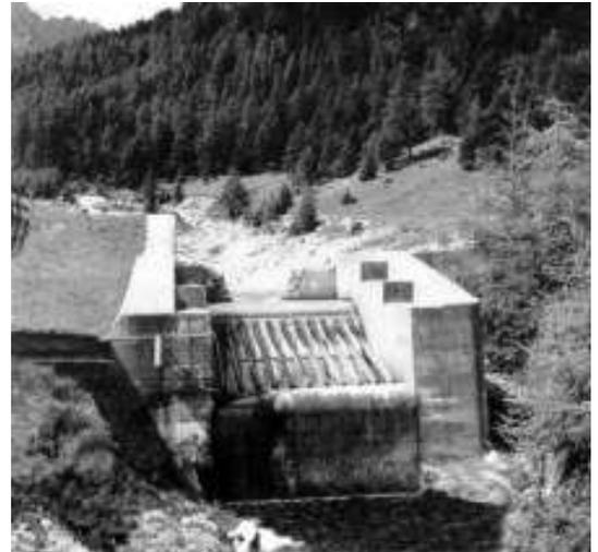
Some bottom intake designs are providing a cleaning bay before the gutter, so that larger rocks and stones get trapped.
