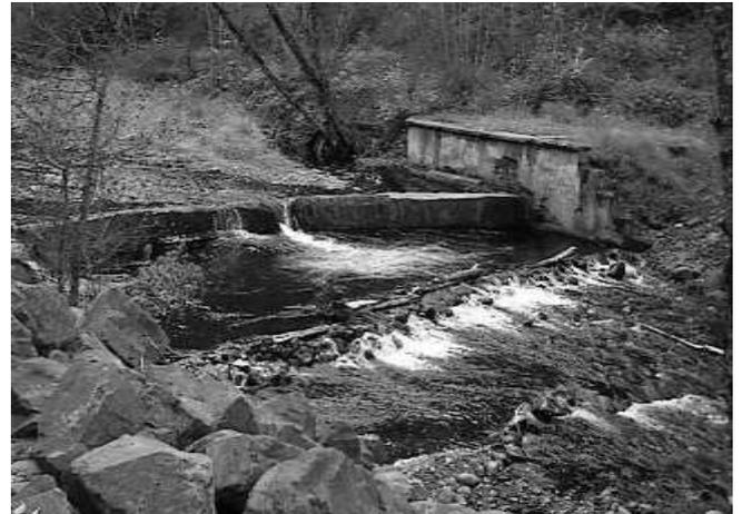
Cleaning the gutter at regular intervals, especially after every heavy rainfall is essential, so that the water flow to the intake is not blocked by logs and other debris.
