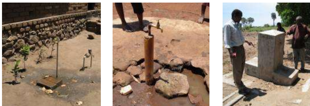
Figure 12 Working household tap, broken rural tap and disconnected community tap
