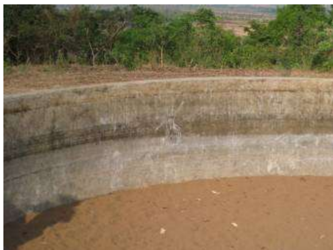
Figure 6 Dry Treatment Plant in Dombole
