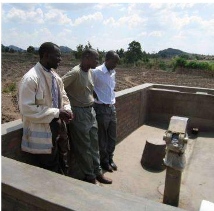
Figure 9 Repaired vandalised pump
