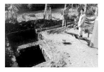
*Figure 2.5 Well proportioned mud pits ready for filling*
