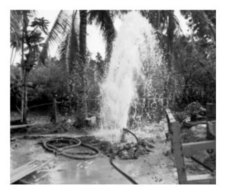
Figure 7.12 Final stages of developing with compressed air
