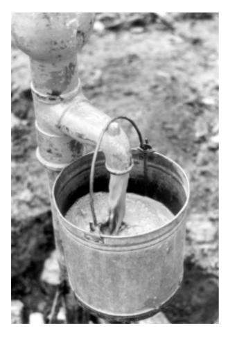
Figure 9.2 Borehole inadequately developed and left for user to sort out
