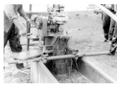
Figure 3.2 Drilling with compressed air – having "struck" water
