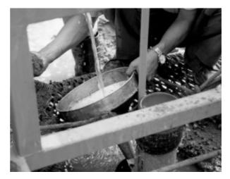
Figure 7.19 Gravel packing – note water flow up has stopped – gravel landed abobe screen level
