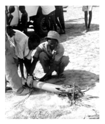
Figure 7.2 Heating up pipe end to form points
