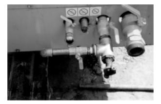
Figure 7.11 Air development manifold – Allowing discharge to atmosphere
