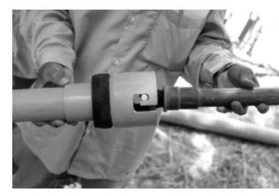
Figure 6.10 Placement of telescopic screen using simple bayonet tool
