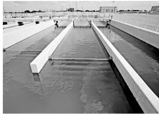
Figure 11-20 Baffling in chlorine contact basins: (a) placement of baffles in chlorine contact tank at the beginning of each channel (or pass) is critical (adapted from Crittenden et al., 2005), (b) typical submerged baffle detail (adapted from Kawamura, 2000), (c) effect of the use of baffles in chlorine contact basins (adapted from Hart, 1979), and (d) view of chlorine contact tank with submerged wooden baffles placed at the beginning and end of each channel.
