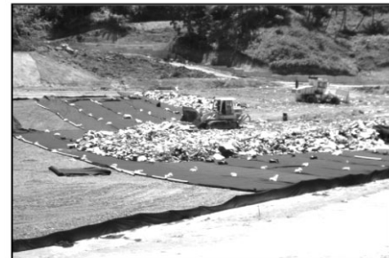
Sanitary landfill under construction, St. Lucia (Courtesy: C. Jules)
