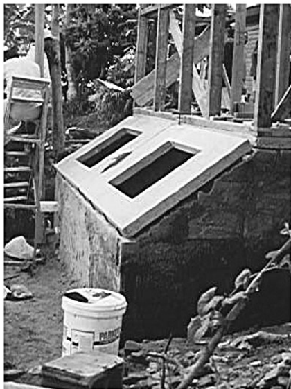
Construction of composting toilet in Fiji (Courtesy SOPAC).
