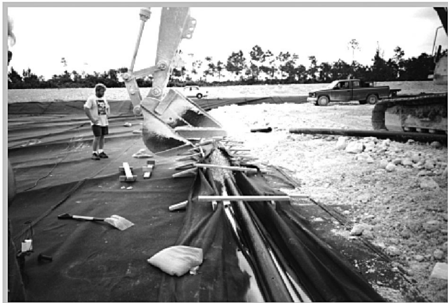
Sanitary landfill synthetic lining being installed, Bahamas (Courtesy: H. Sealy)
