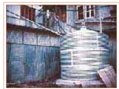
A storage tank made of galvanized iron sheets
