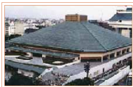
At Kokugikan sumo wrestling arena in Tokyo, Japan, rainwater collected from the arena's 8,400 square meter rooftop is used for non-potable purpose.
