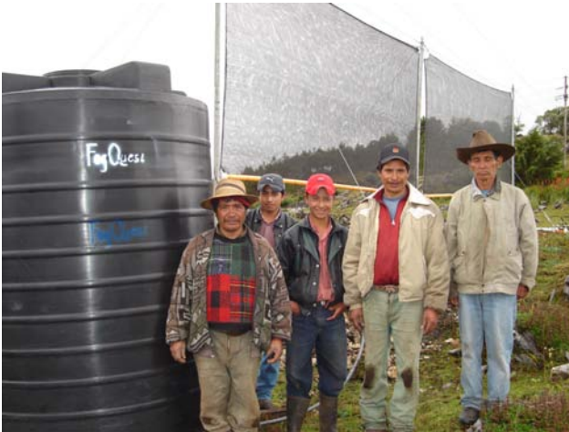
Figure 5: FogQuest Project, Tojquia, Guatemala, October 2006. Two large fog collectors and one 3000 liter tank provide water for one or two families.
