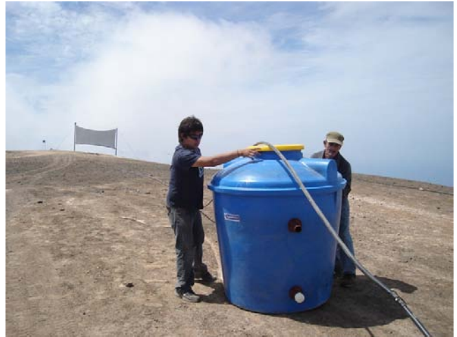
Figure 6: A 1300 liter water tank and fog-water pipeline, Alto Patache, Atacama Desert, Chile.
