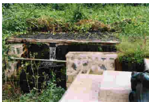
A protected spring in eastern Zaire being used to supply two large refugee camps
