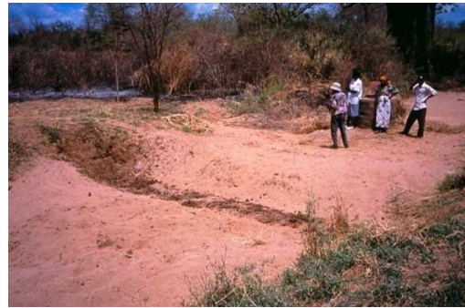
One of the subsurface dams built of soil at Kibwezi, Wote and Matiliku in 1992-96.
