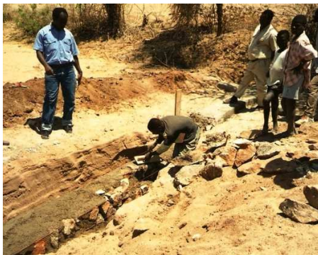
A subsurface dam being built of rubble stone masonry and an old well. Dodoma 1990
