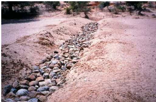
A subsurface dam built of soil and covered with stones at Dodoma in 1990.
