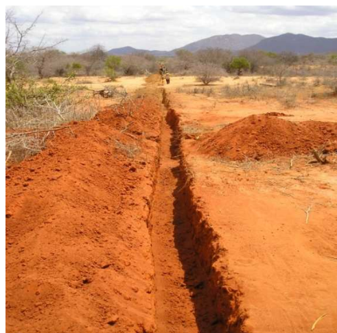
An excavated trench for pipes.
