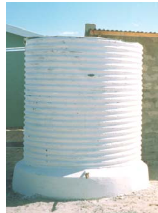
A repaired tank.
