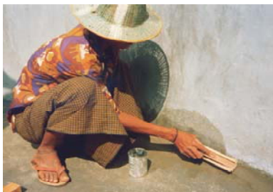
An internal apron can be made with a short length of bamboo
