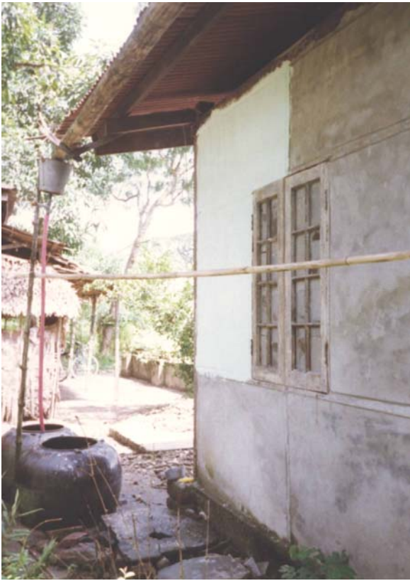
Water from a gutter made of a split bamboo is delivered to the jars by a bucket and a hosepipe.
