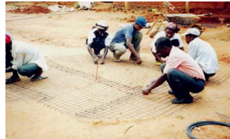
Weld mesh cut to fit
