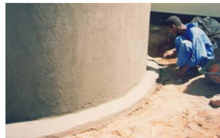
An external apron is made with a or an empty beer bottle.
