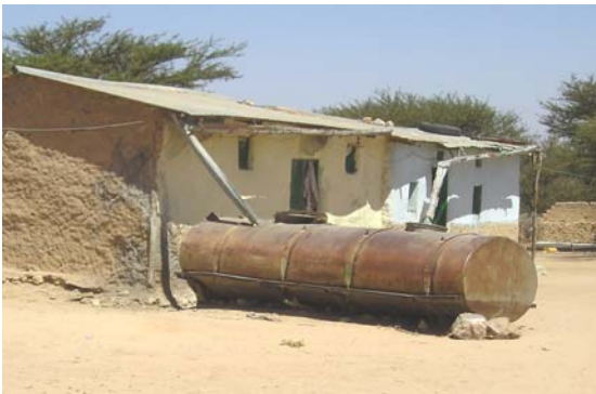
A discharged petrol tank used for roof catchment of rainwater in Somaliland.
