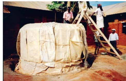
A newly plastered tank must be
