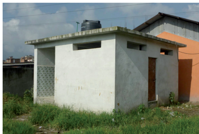
Figure 6: The toilet building at the Kuleshwor Secondary School in Kathmandu. Urine is collected in tanks (see below).
