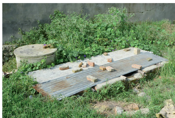
Figure 7: The collected urine is conveyed to two underground tanks. The soak pit in the back absorbs overflowing urine.
