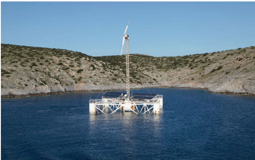
Fig. 13.24 Hydryada, a floating desalination unit in Irakleia, Cyclades, Greece, powered by wind and solar energy
