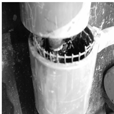
Figure 3.9: Modified outlet of the ABR showing mesh for preventing coarse solids entering the flow meter.
