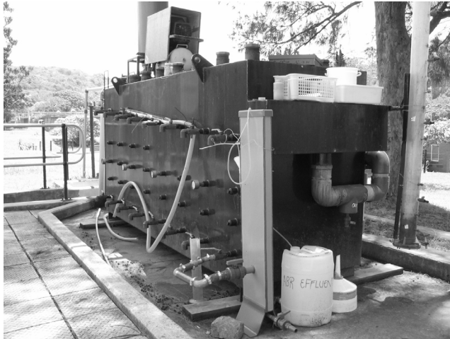
Figure 3.8 Installation of the ABR at Kingsburgh WWTP. The outlet end of the pilot ABR showing the membrane unit attached to the last compartment (left); and a laundry basket housing the submersible pump in a wastewater sump near the feed end of the ABR (right)
