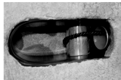
Guide box cast in concrete
