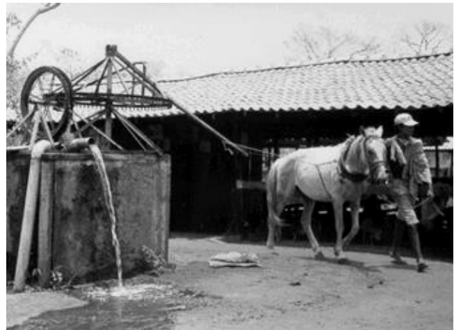
Animal powered Rope Pump
