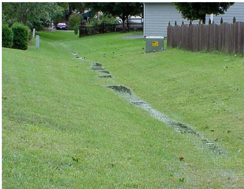
Grass Swale through residential area. Note flat slope to encourage infiltration – ponding water gone within hours of runoff producing event.
