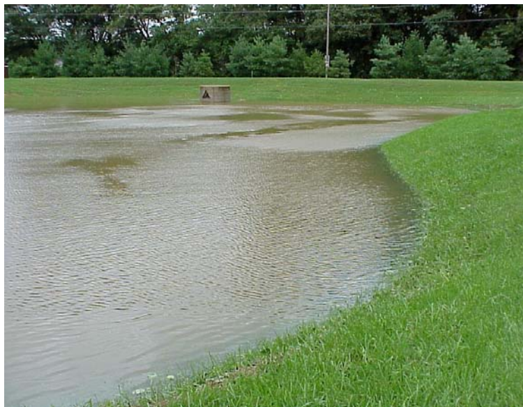
Extended Detention Basin – full.
