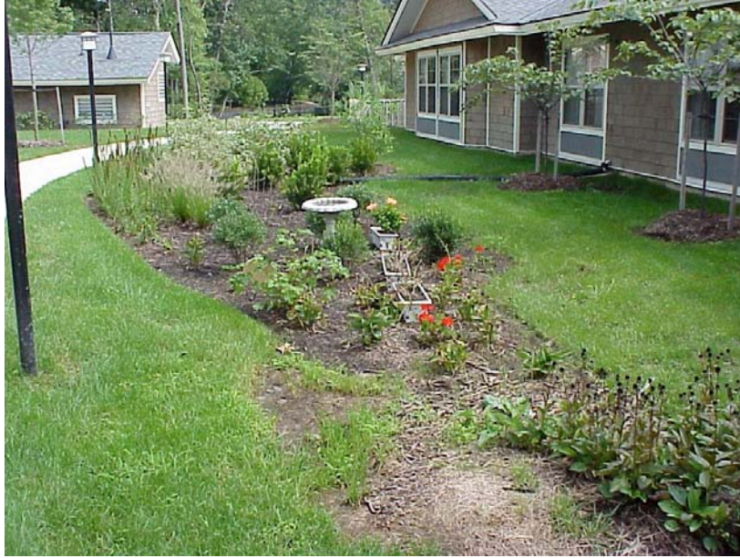
Bioretention Filter in multi-family residential setting.
