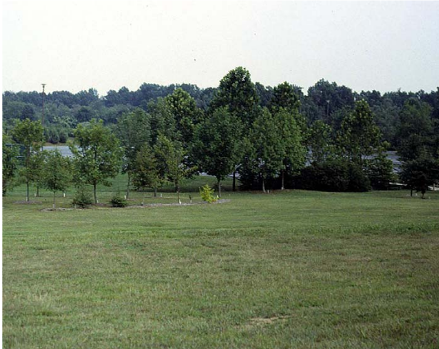
Vegetated Filter Strip. Note landscaped areas parallel to contours to force runoff to spread out. No evidence of channel flow short circuiting filter strip.
