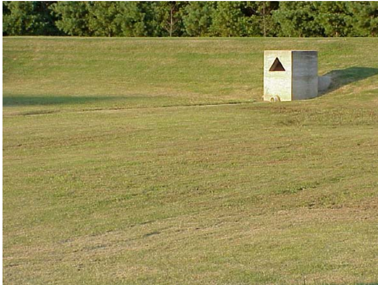
Extended Detention Basin – empty.
