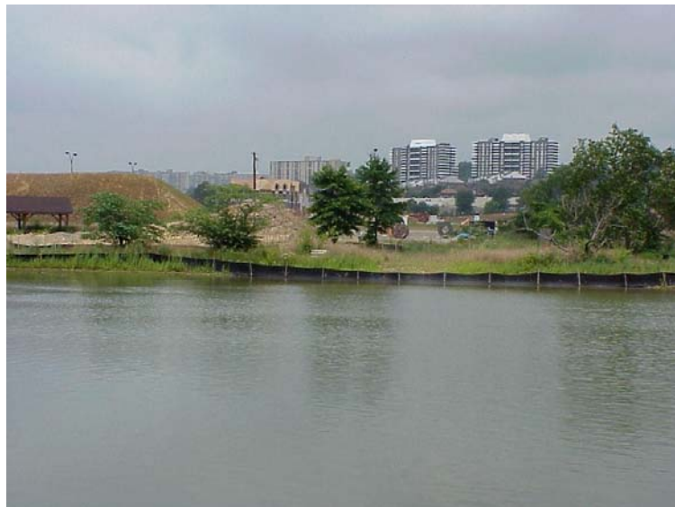
Retention basin in ultra-urban setting (under construction).
