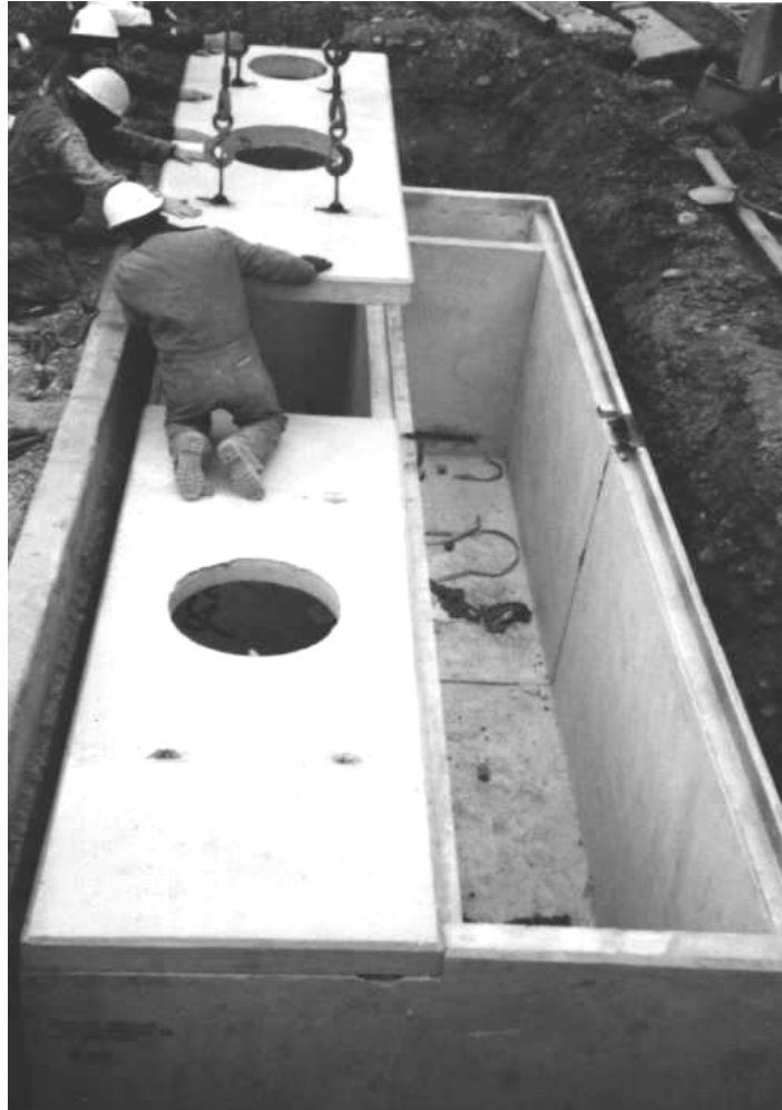
FIGURE 3.12B - 3 Installing Precast Delaware Sand Filter Shell in Alexandria, Virginia
