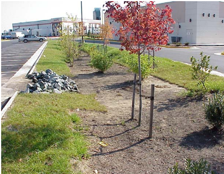
Bioretention Filter located in required parking lot green space.
