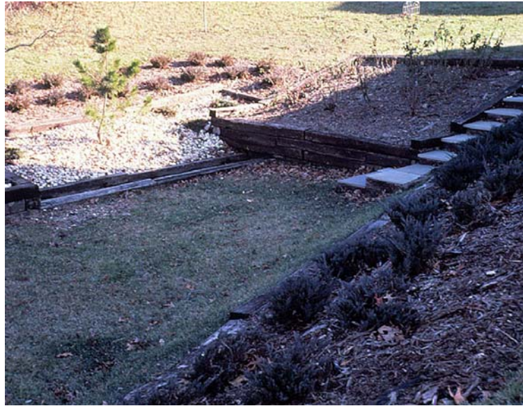
Infiltration Basin serves as landscaped pedestrian area during dry periods.
