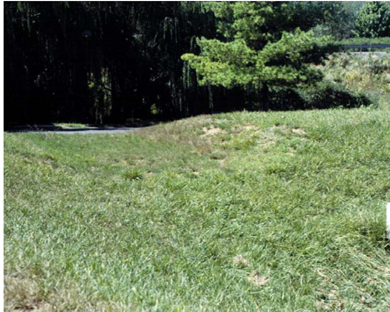
Emergency Spillway “cut” into existing grade.
