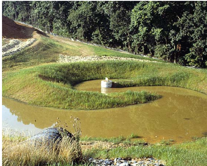
Extended Detention Basin – full. Note circuitous flow path.
