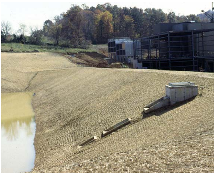
Stabilization of newly constructed Earthen Embankment
