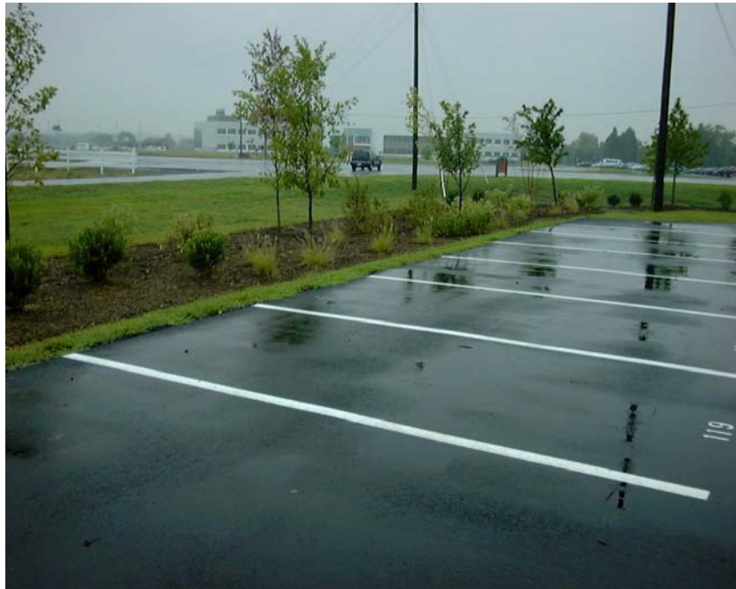
Bioretention Basins in office setting parking lot.
