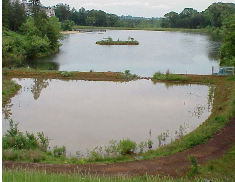
Sediment Forebay constructed with earthen embankment and rip-rap overflow.
