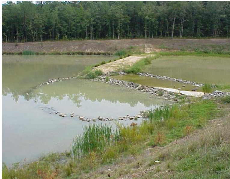
Sediment Forebay constructed with submerged rip-rap weir.
