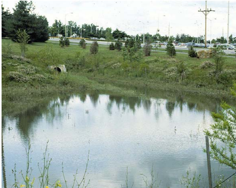
Landscaping – “rough” shoreline edge and aquatic bench provides improved pollutant removal and shoreline stabilization.
