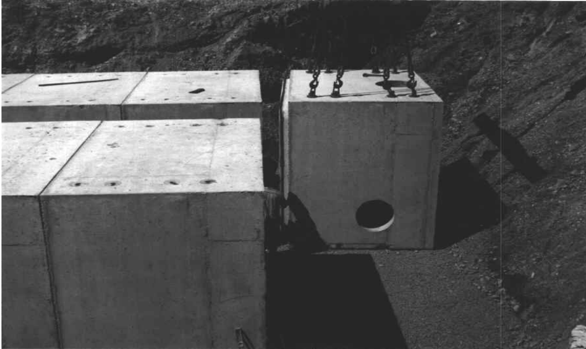
FIGURE 3.12A - 4 Installing Precast D.C. Sand Filter Shell in Alexandria
