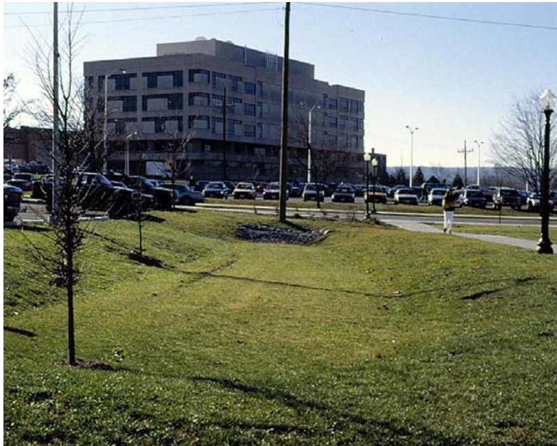
Grass Swale. Note stone check dam in front of inlet creates shallow ponding area to encourage infiltration and settling.
