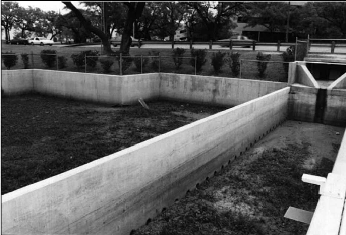
FIGURE 3.12 - 1 Austin Partial Sedimentation Surface Sand Filter
