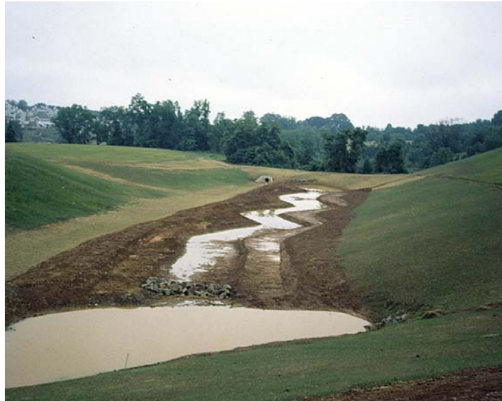
Constructed Stormwater Wetland – recently completed.
