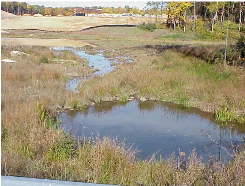
Forebay and Constructed Stormwater Wetland incorporated into regional retention basin design.
