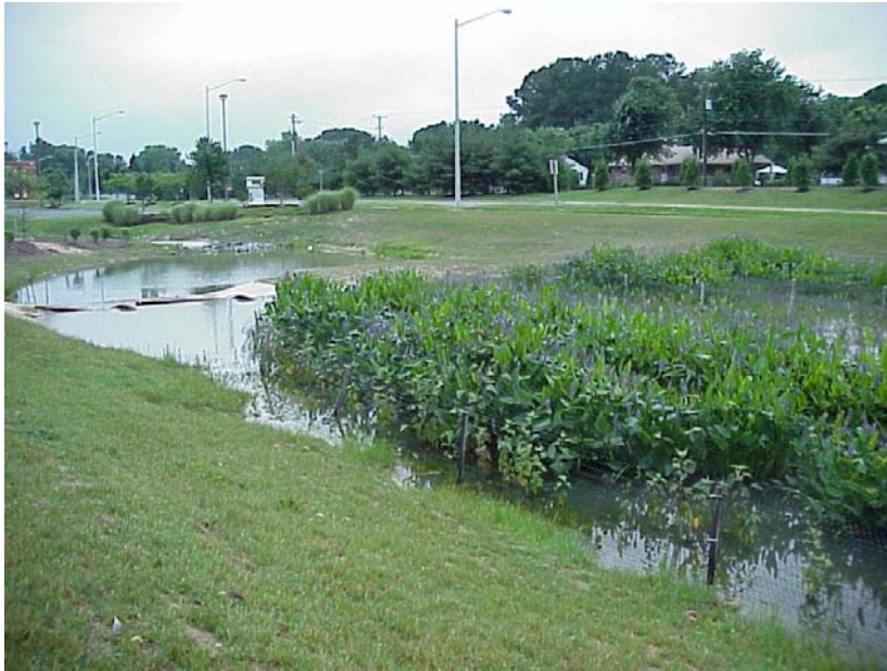
Constructed Stormwater Wetland. Note vegetation protected from waterfowl by netting system.
