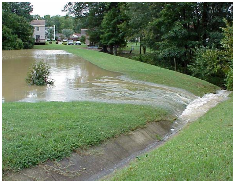
Emergency Spillway draining into concrete channel to protect embankment from erosion.
