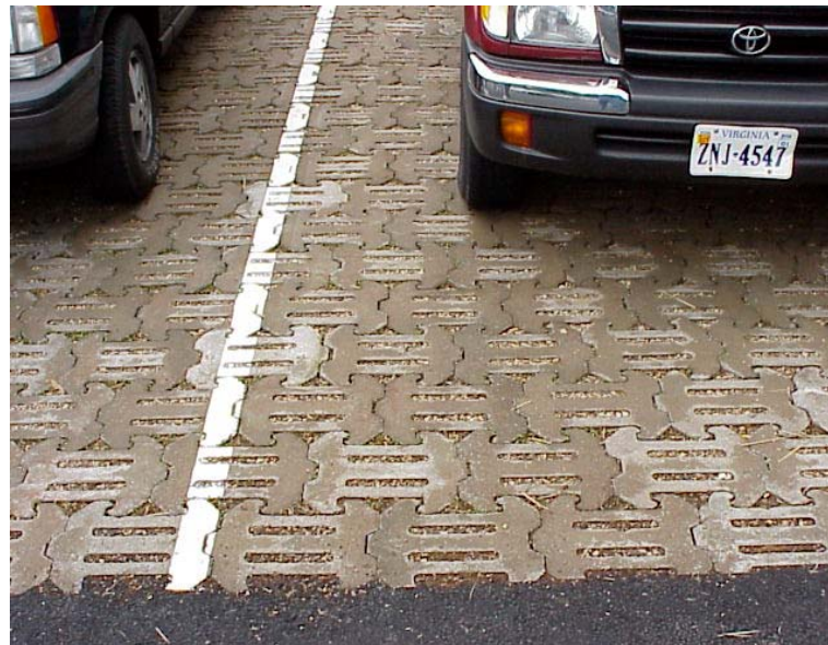
Infiltration Trench with concrete parking pavers in office park setting.
