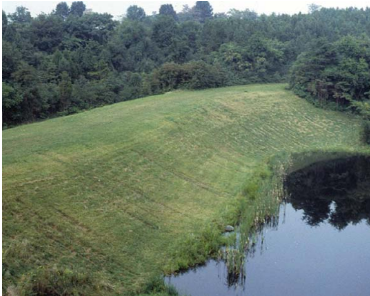
Typical Earthen Embankment
