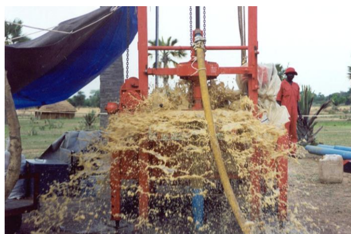
Figure 5: Well Development using Compressed Air
