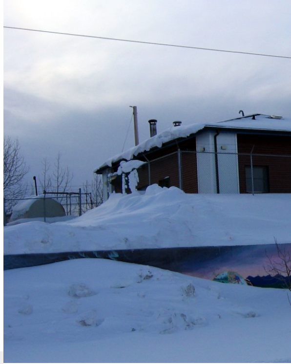
Mechanical Treatment Facility Building
