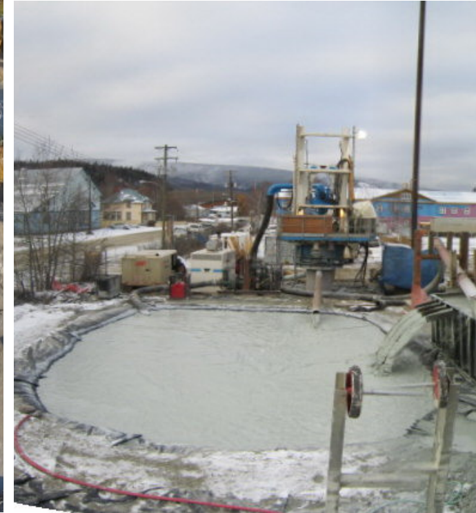
Drill mud recycling for construction of two 100 deep shafts
