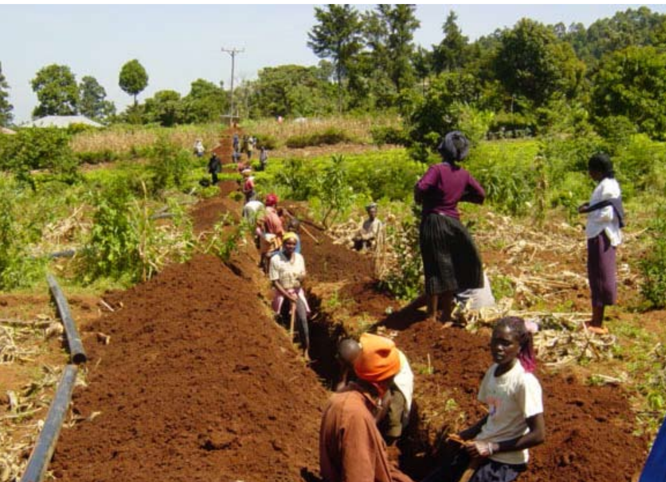
Community joint effort in digging trenches for water pipes. Photo © UN-Habitat
