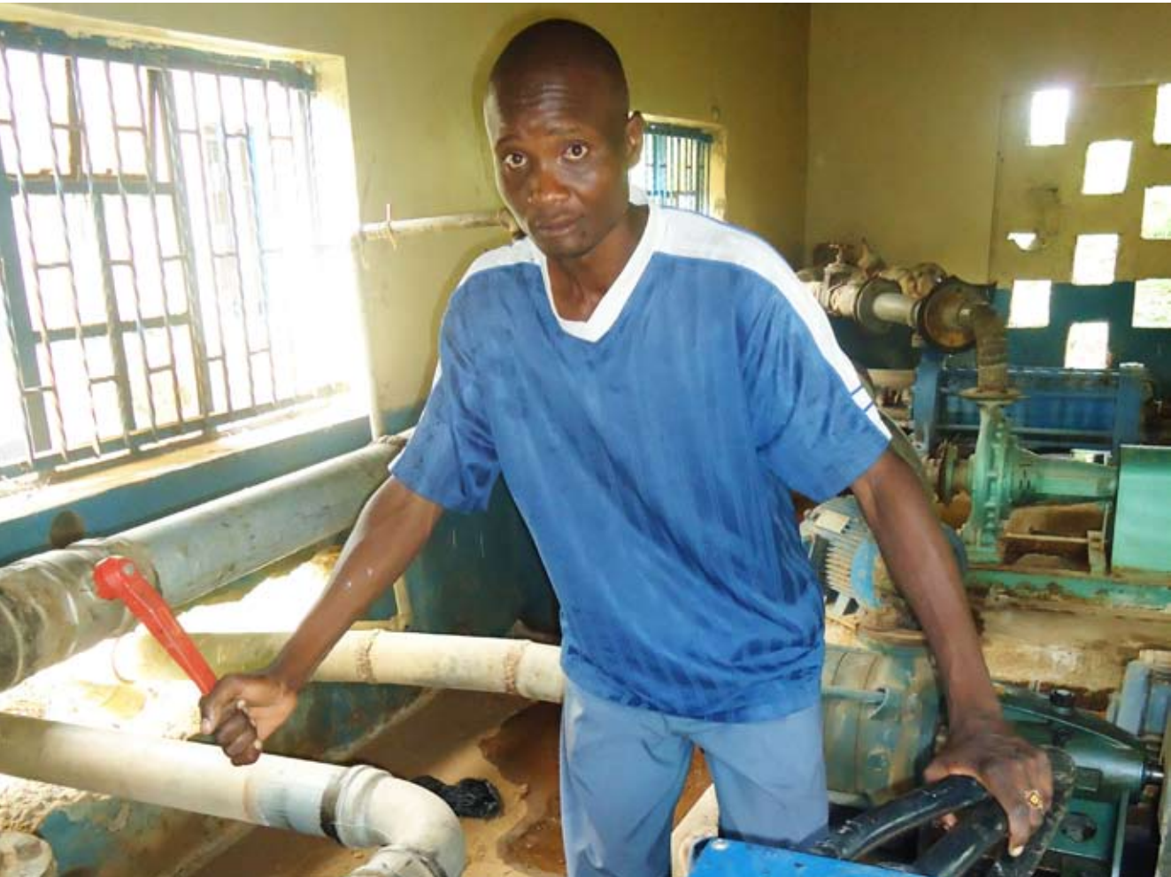
Repairs in the water pump house. Photo © UN-Habitat
