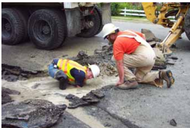
Mike Carlstrom, Tacoma Water construction inspector, tackles a distribution system leak. Tacoma Public Utilities Photo
