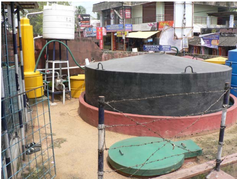
Figure 5: Different types of BIOTECH biogas plants. Top middle: a) 1 m 3 domestic level plant for the treatment of kitchen waste. Top right: b) 2 m 3 domestic level plant with a link for a toilet and an inlet for kitchen waste. Top left: c) 4 m 3 institutional level plant. Lower left: d): 25 m 3 market level plant equipped with gas scrubber and generator (Pictures: Florian Heeb).
