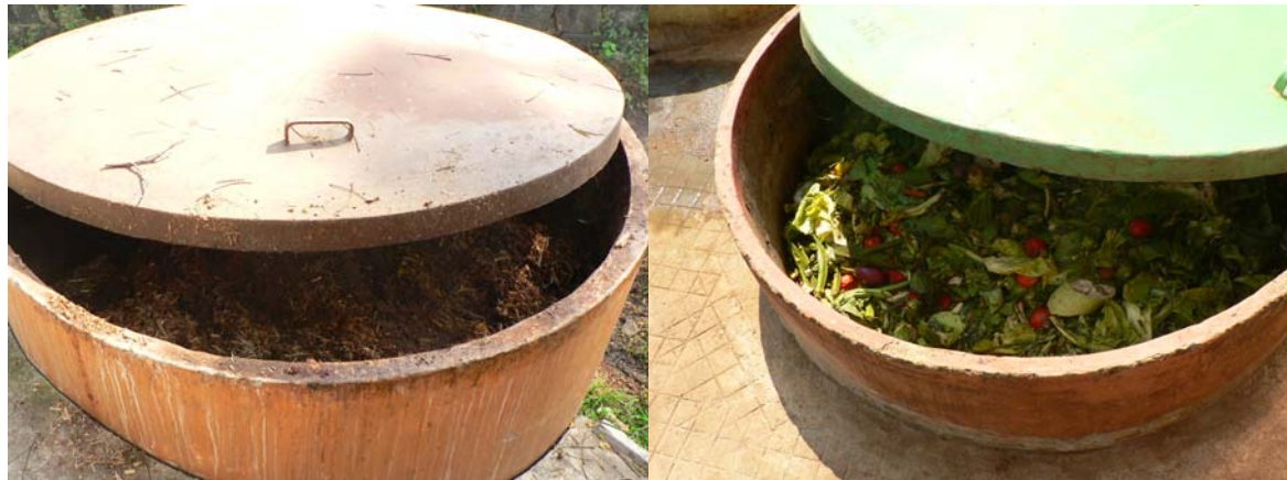
Figure 11: Pre-digesters filled with vegetables (left) and with pre-digested fibrous material (right) at the Govt. Ayurveda College, Trippunithura and at the market of Thrikkarakara, respectively (Pictures: Florian Heeb).
