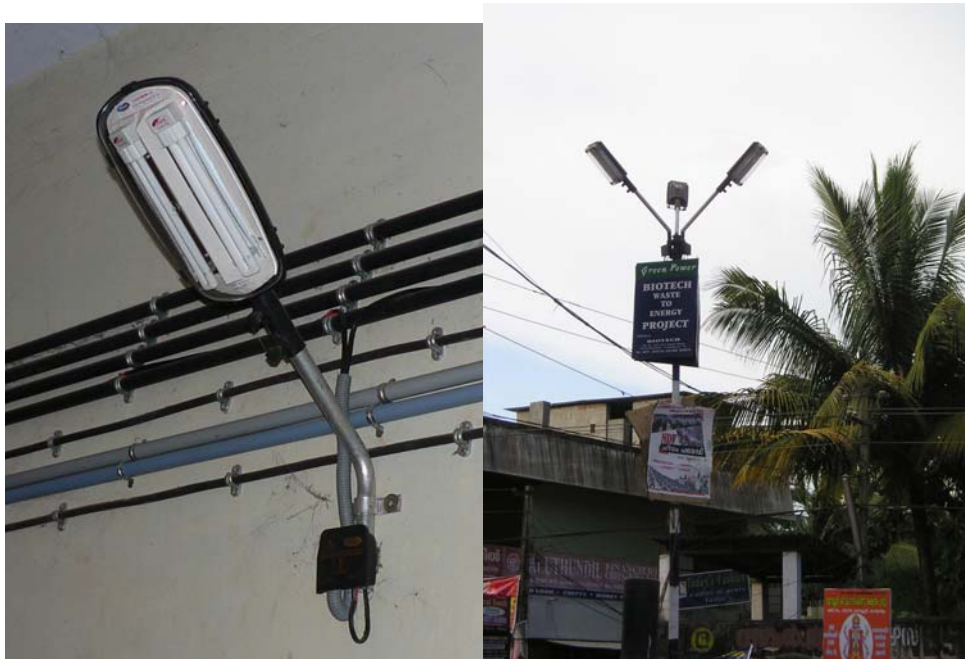
Figure 7: Chemo fluorescent lamp installed by BIOTECH at the Govt. Ayurveda college, Trippunithura (left) and at the market of the Sreekaryiam Grama Panchayat (right). The lamps consist of two 11W bulbs (left picture: Florian Heeb; right picture: Christian Müller).
