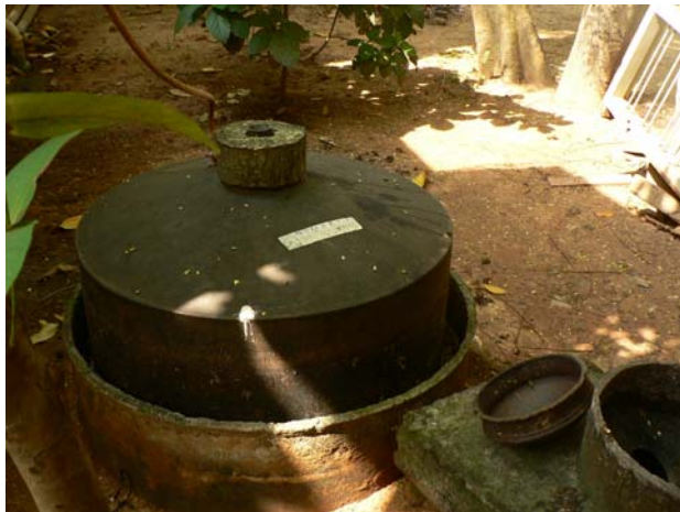
Figure 3: BIOTECH domestic plant with ferro-cement digester tank. The plant has been in use for ten years, problems have occurred only very rarely (Picture: Florian Heeb).
