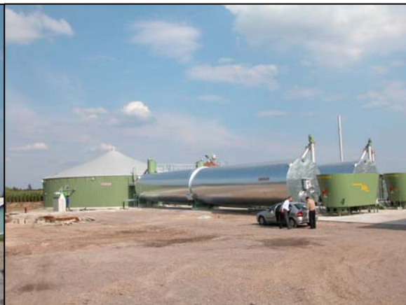
Figure 5. Horizontal Digester
