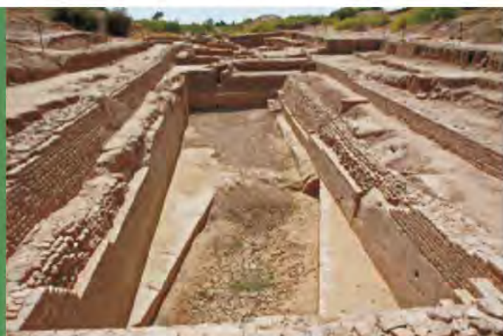
Fig. 1.1 : The stone bunds erected at Dholavira (Harappa Civilisation) forming a reservoir to conserve rainwater. Source: [Accessed: 10.07.2013]. http://www.shunya.net/Pictures/WesternIndia/Gujarat/Dholavira/Dholavira03.jpg
