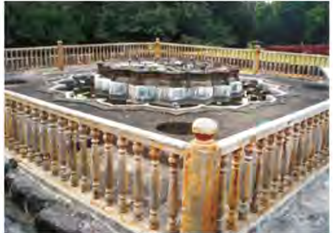
Fig. 1.4: The Hajari Karanje (thousand outlet fountain) in the historic Shaniwarwada Fort. This fountain received water through underground aqueducts directly from the Katraj Lake 10 km away. [Accessed: 10.07.2013] Source: http://travelzunlimited.blogspot.in/2010/11/shanivar-wada-pune-photo-feature.html
