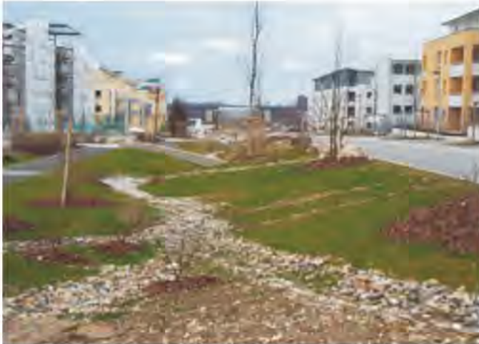
Fig. 2.2: Natural system for managed stormwater collection, treatment and infiltration in Switzerland. Source: Heeb 2008
